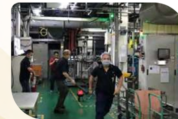
Fire Discovery - Initial Firefighting
